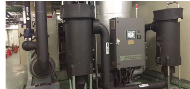
[ASE Chungli] Adjustment of air compressor
